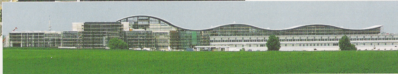
Building site of Greifswald Branch Institute of IPP
